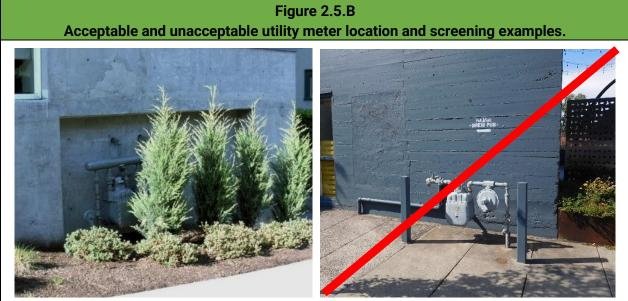
Place utility meters in less visible locations. The left examples is successfully tucked away in a less visible location and screened by vegetation. The right image is poorly executed and would not be permitted in such a visible location; such meters must be coordinated and better integrated with the architecture of the building.
