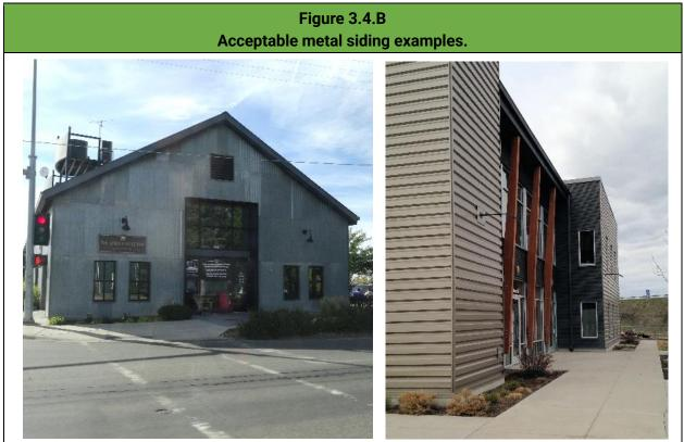
Left: A metal wall with roof overhang is acceptable; the lighting and wall opening framing also help improve the façade composition. Right: A good departure example without a roof overhang, but the short length of the walls, amount of window openings, and color/pattern changes create an acceptable design that meets the intent of the standards.
