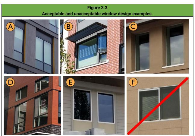
The windows in Images A-C are recessed by at least two-inches from the façade. Images D and E feature a reveal/recess of less than two-inches, but the contrasting frames and mullions effectively add a sense of depth and richness to the façade. The treatment in Image F does not effectively meet the design criteria.
