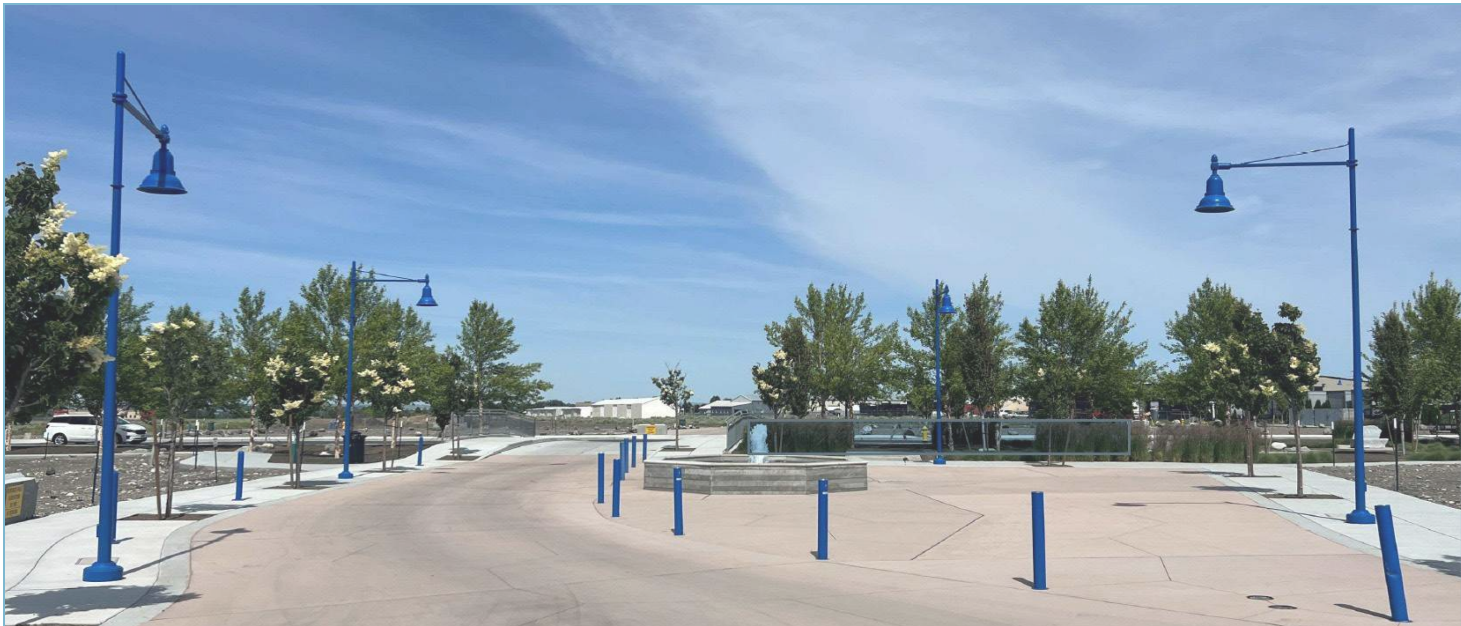
VISTA FIELD METAL AREA LIGHT AND BOLLARDS
