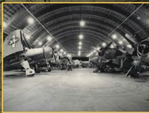
Drill Hall hangar at Naval Air Station Pasco on September 18, 1944. Aviation cadets assigned to the base trained in Pasco and at Vista Field.
