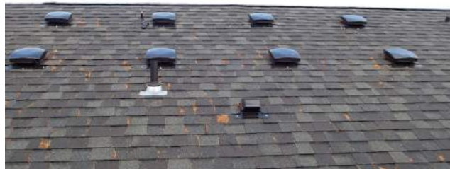
Roof vents – the wrong way!
