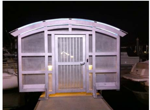
New marina gates installed by Ray Poland & Sons.
