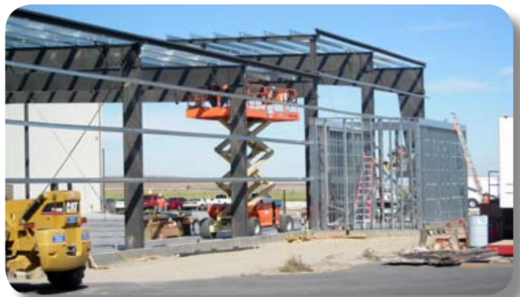
Construction underway at Pacific Rim Winemakers.
