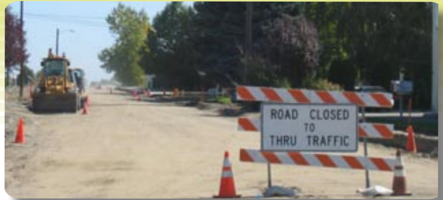
Fowler Street Construction
